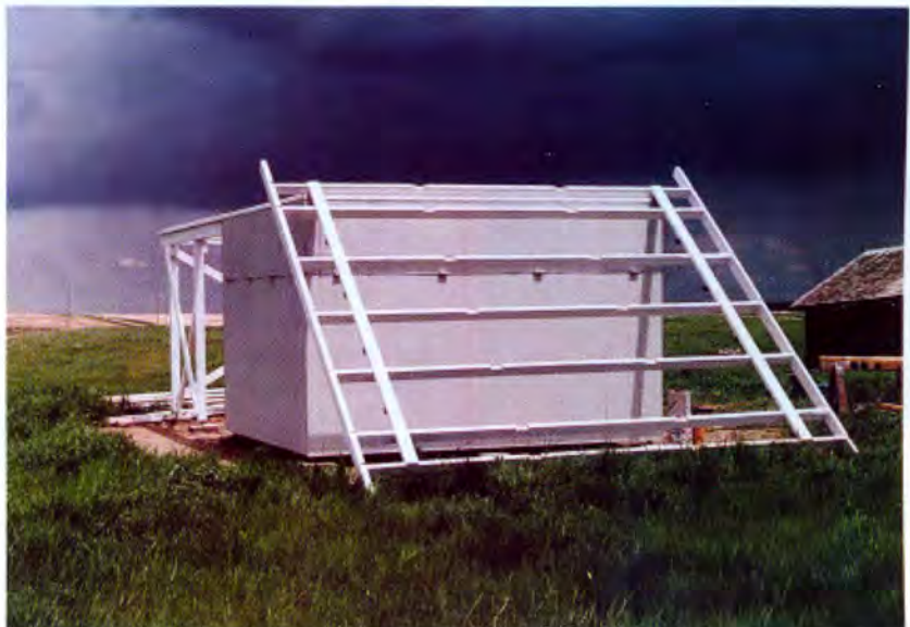
THE ROLLING FRAME was reassembled at the observatory on the ground and lifted into position (below). One-inch aluminum angle, screwed every 12 inches along the length of the rails, guides the frame's casters when rolling the roof back and forth (left).
