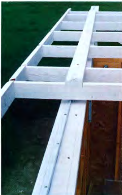
THE ROLLING FRAME was reassembled at the observatory on the ground and lifted into position (below). One-inch aluminum angle, screwed every 12 inches along the length of the rails, guides the frame's casters when rolling the roof back and forth (left).
