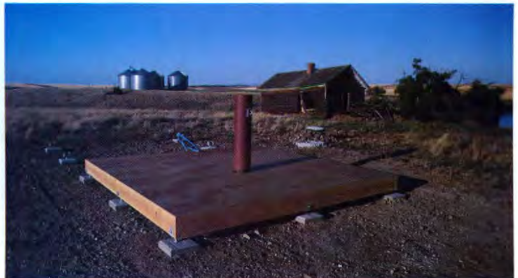
THE FLOOR IS FRAMED with 2x8 joists on 16" centers fastened to 4x8 rim joists on the west and east walls (above). The perimeter joists are bolted to the post supports cast in the concrete footings. Bridging is installed around the pier to help support the 5/8" plywood subfloor.
